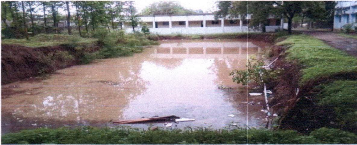
Check Dam Constructed in the campus
